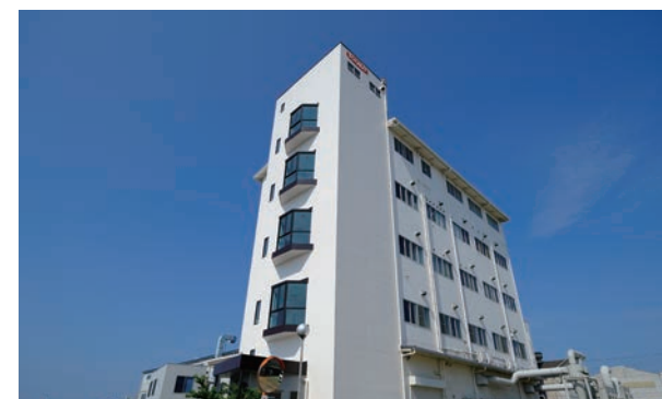
Thermal Spraying Technology R&D Laboratories
